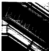
143 Renault Distribution Centre, Swindon, England, 1980–82; slotted-steel escape stairs cast crisp shadows.
